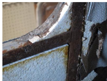
Insulation and metal framing of an older caravan
